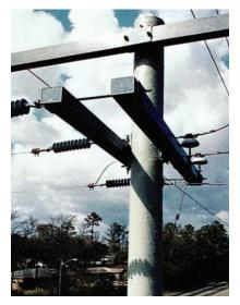
"Owens Coming has solved that problem with their Advantex corrosion resistant E glass fiber that is low in seed count. Insulator manufacturers like MacLean Power Systems can now take full advantage of boron-free glass fibers and also have wicking performance comparable to standard E glass. MacLean Power Systems can now offer the utility engineer that extra margin of safety at a relatively low incremental cost," said Schmiedeknecht.
