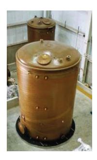
To help its customers avoid corrosion from acidic brine and other harsh chemicals, Michigan-based Belding Tank Technologies, Inc. relies exclusively on boron-free Advantex® E-CR glass from OCV™ Reinforcements.
